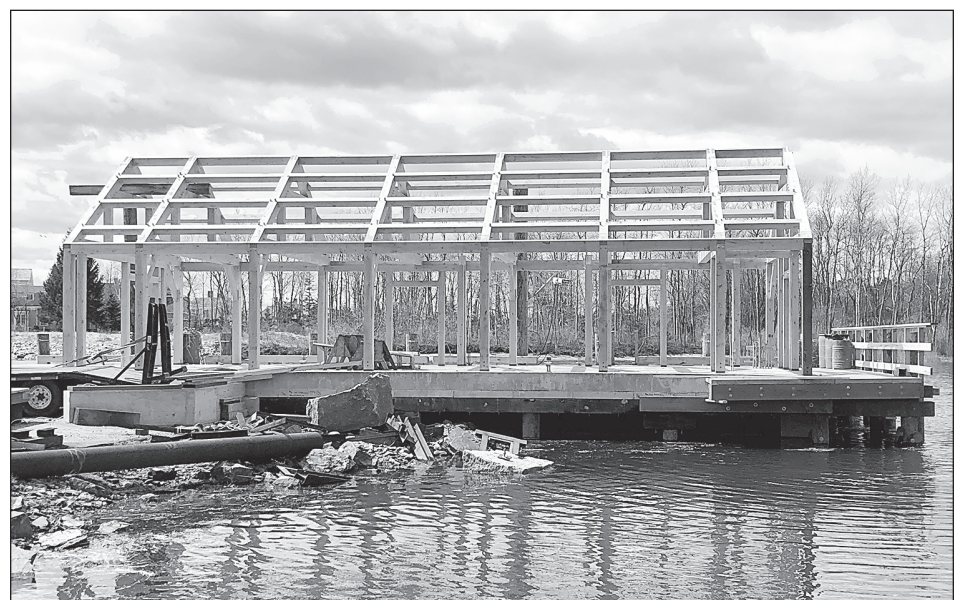
Framing under construction for the new bait shed at Government Wharf.
