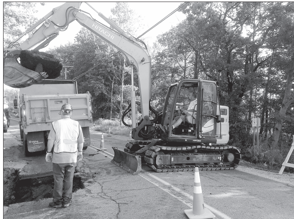
Kevin Paradis of public works excavates a trench on Mills Road for installation of a new drainage culvert.
