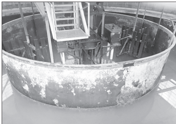
Picture of rotted stilling well in one of the secondary clarifiers.
