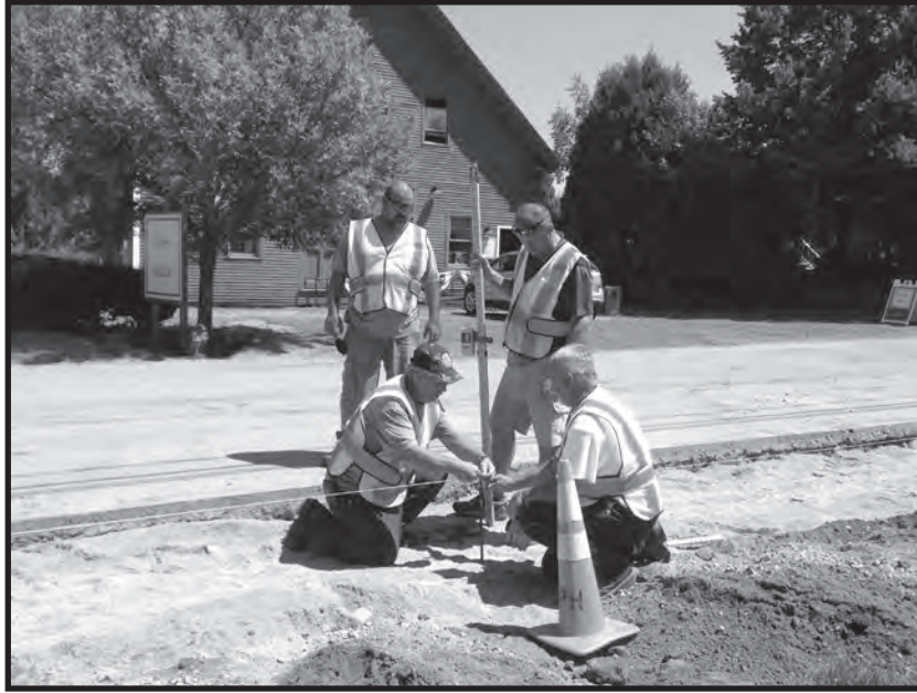
The public works crew installing granite curb for sidewalk on Langsford Road
