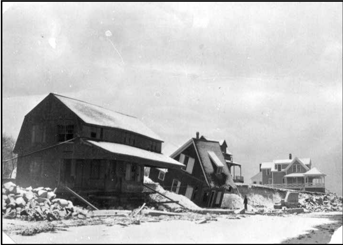
A January 1933 storm caused severe damage to several cottages along Goose Rocks Beach when their seawalls were destroyed.
