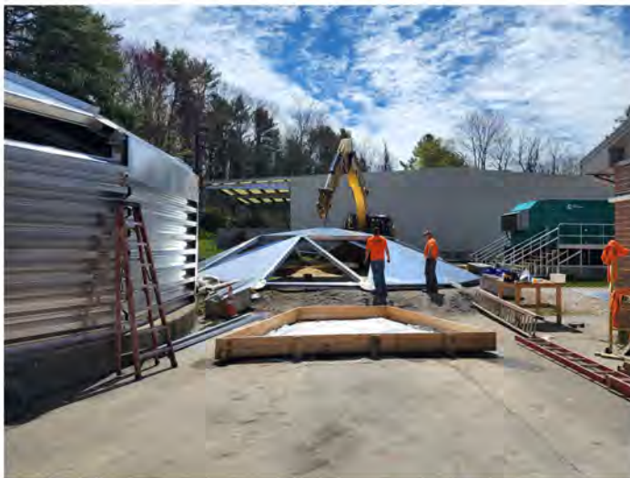
Putting the finishing touches on the new clarifiers
