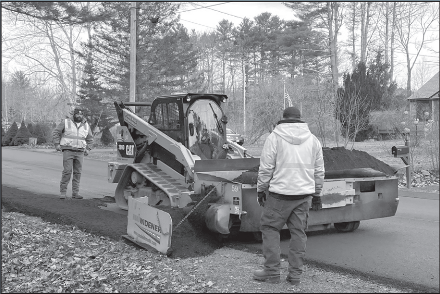
Shoulder work being completed with the use of the CAT Road Widener.
