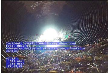
MSA - Survey Abandoned @ 79.8 ft. bottom of pipe is gone, unsafe to continue
