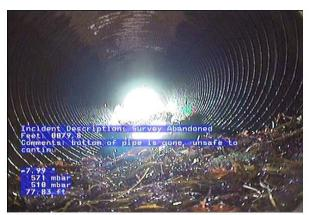
MSA - Survey Abandoned @ 79.8 ft. bottom of pipe is gone, unsafe to continue
