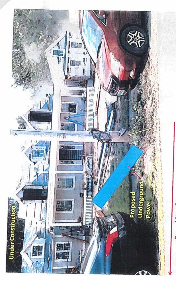
Pave sidewalk cut and pave sidewalk from cut to end of sidewalk 3/4 " overlay By Home Owner.
